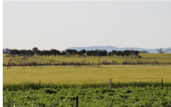
Progressive failure of Transmission lines occurred in South Australia during Sept 2016 Thunderstorms.
