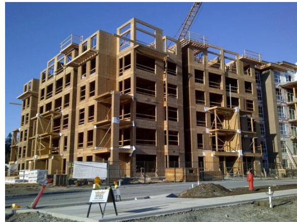
Multi-story wood framed building
